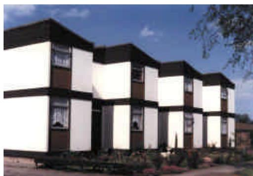
**Figure 14** Calder houses. *One of the better known forms of Volumetric housing*
