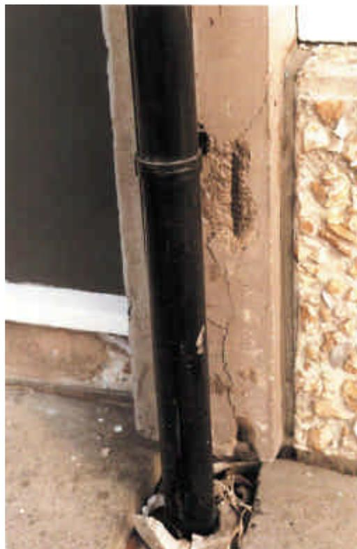
**Figure 12** Shepard Spacemaker LPS building with extensive cracking and spalling in exposed ends of cross walls
