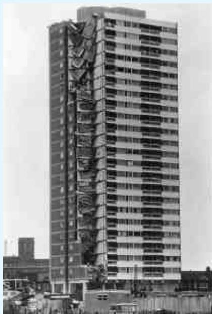
**Figure 6** *Ronan Point following collapse*
